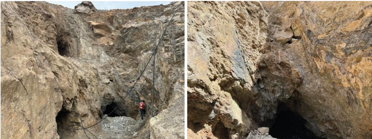
Figure 34. Previous mining work.
